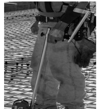
Fig. 2: Rebar tying using power tier with extension handle
