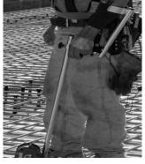
Fig. 2: Rebar tying using power tier with extension handle
