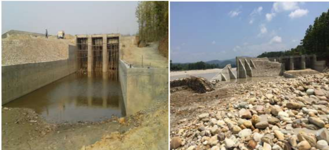
Fig. 1: Completed Part of Badkpath Intake Fig. 2: Damaged Intake after the flood
